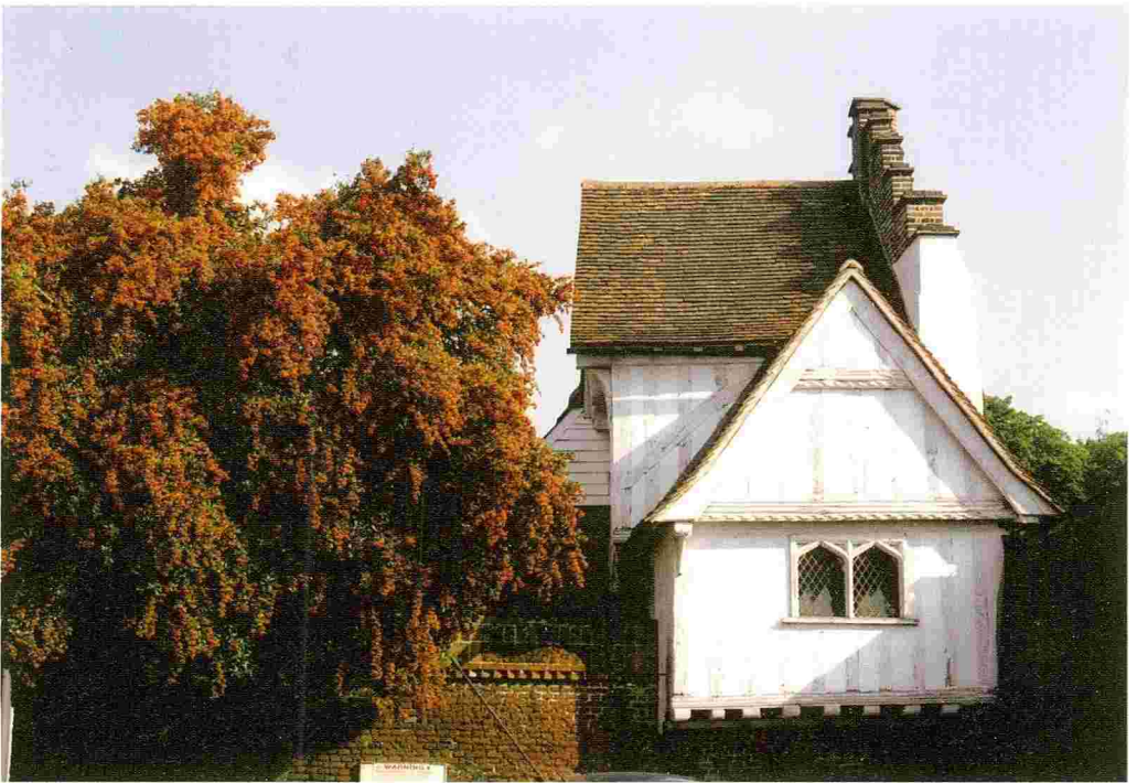
FIG. 72 – Ipswich, Suffolk. Former archdeacon's residence. View of gatehouse from south. Note the prominent half-timbered extension, c. 1500.
