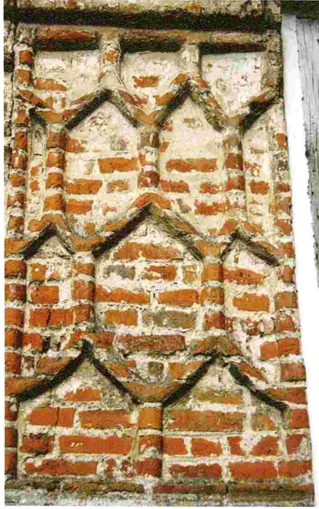
FIG. 73 – Lidgate, Bury St Edmunds, Suffolk. Suffolk House. Carved or moulded brick diapered strapwork on side of end gable facing south-west.
