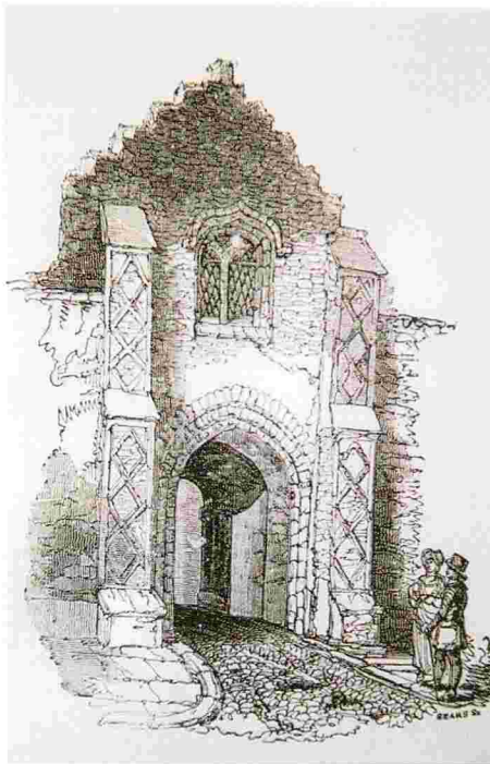
FIG. 70 – Ipswich, Suffolk. Former archdeacon's residence. View of gatehouse from east. Engraving after Sears, 1830. From G.R. Clarke, The History of Ipswich , Fig. before p. 353 (courtesy of Suffolk Record Office, Ipswich). Photo: Tony Hill.
