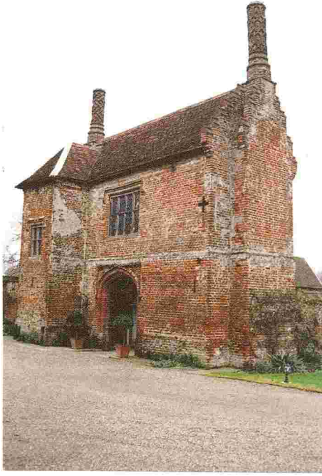
FIG. 86 – Cockfield Hall, Yoxford, Suffolk. Gatehouse. View from south.
